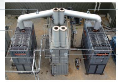
Pipework transferring 469°C exhaust gasses from Generator 2 to the Heat Recovery Boiler.
